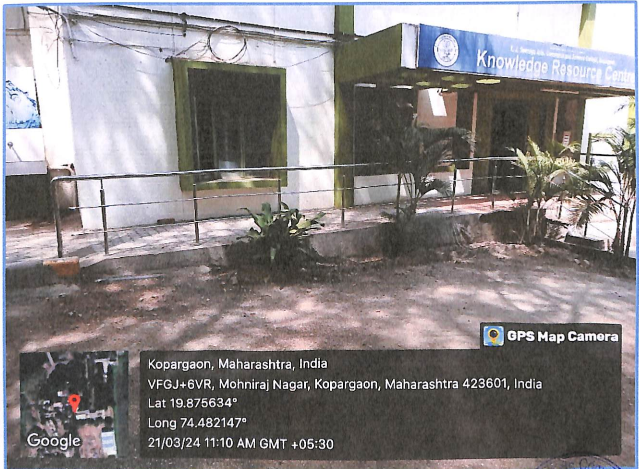
Ramp and Rail at Library Buliding
