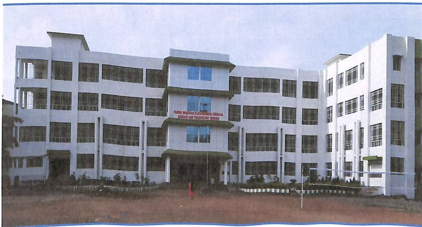
Rain Water Harvested on the Roof of Science Building
