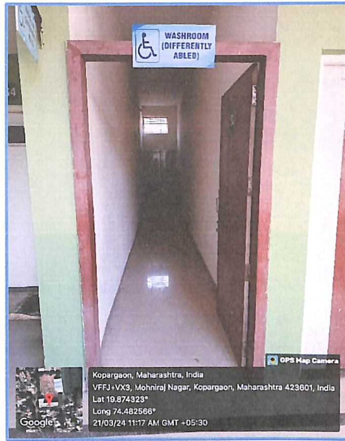
Signage Board at Washroom
