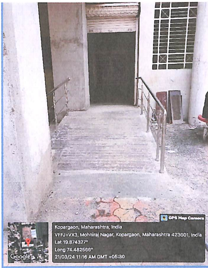
Ramp at Science Building Entrance
