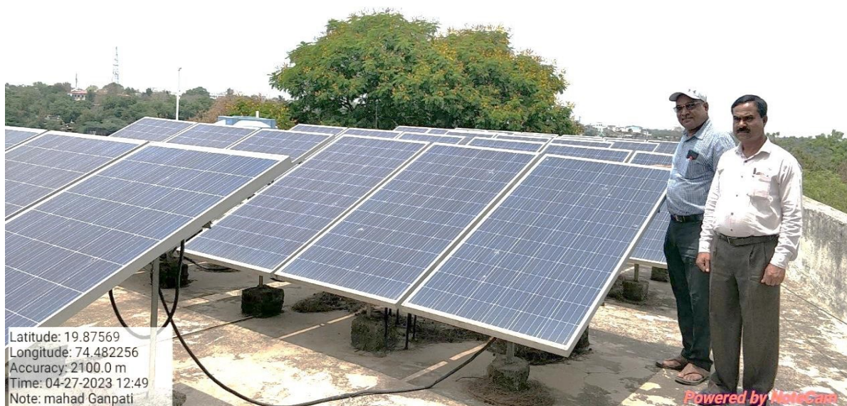
10kW Solar PV system installed on roof top of Library Building
