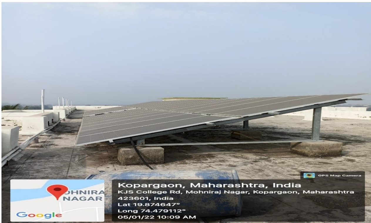
10kW Solar PV system installed on roof top of Science Building
