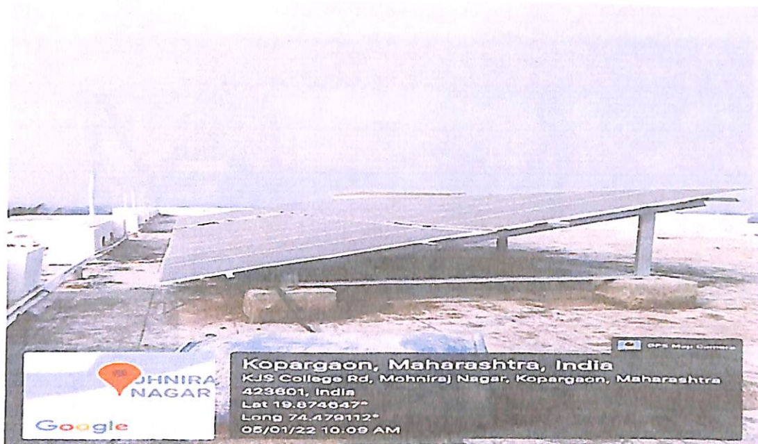
10KW Solar PV system installed on roof top of Science and Technology building.
