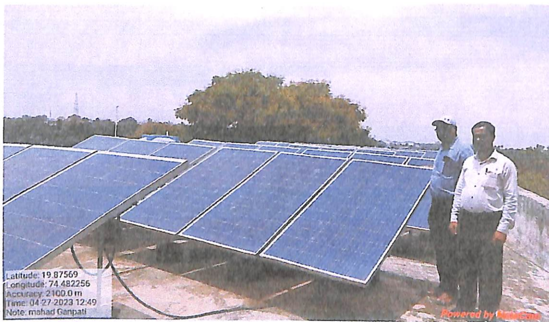
10KW Solar PV system installed on roof top of Library Building.
